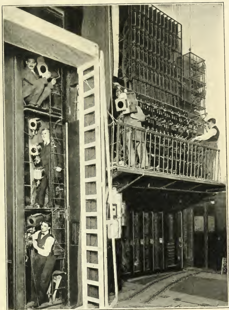
The Electric Switchboard of the Belasco Theatre, the Largest in America
